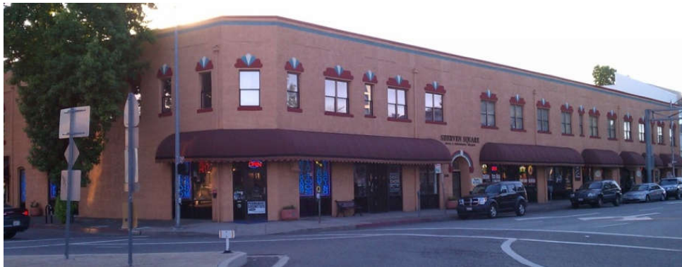
The Giubbani Building (now Sherven Square) today.
