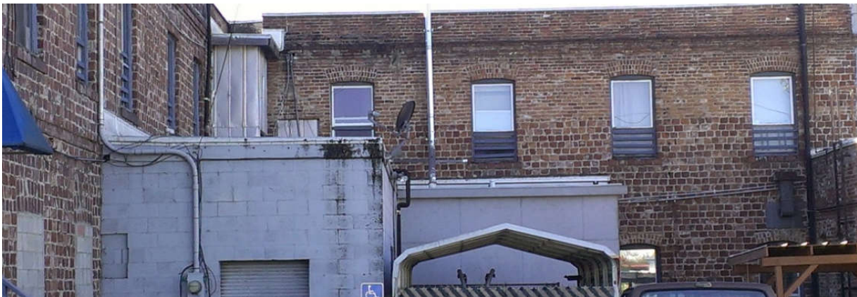
Rear of building, from Taco Bell parking lot
